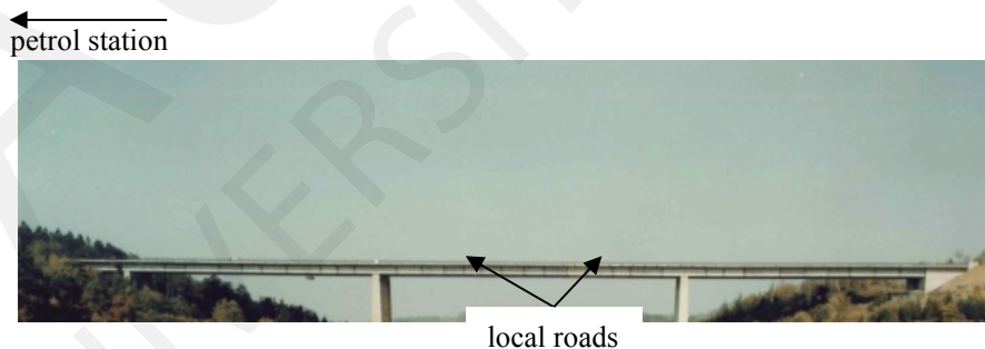
Figure 3: Highway bridge over a wide and deep valley.
