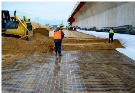
(b) flexible abutment
