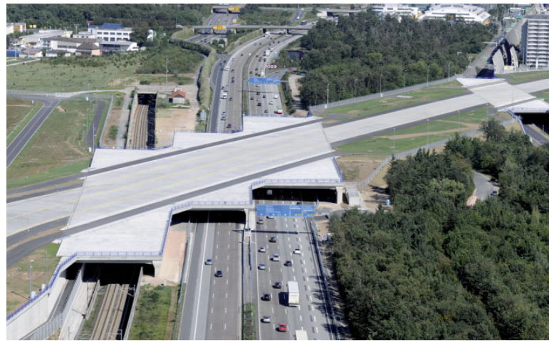
(a) completed bridge
