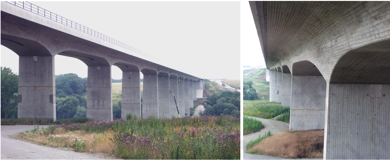
Figure 3.50: Semi-integral “Viaduct Scherkondetal”
