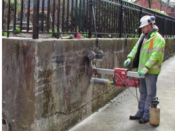
Figure 2. Destructive testing (core sampling)
