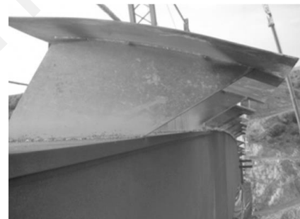
Figure 5. Detail of Deflectors [Corriols A., Morgenthal G. (2012)].
