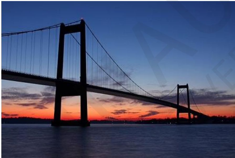
Figure 1. Lillebaelt suspension bridge, Denmark [ http://www.phosee.dk ]
