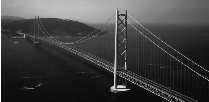
Figure 1.2: Akashi-Kaikyo Bridge, Japan [5].
