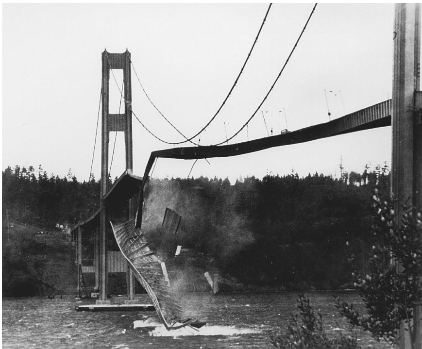
Figure 1.1: The original Tacoma Narrows Bridge collapse, USA [3].
