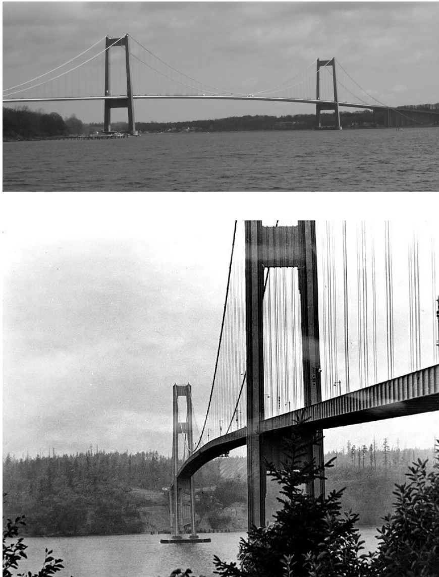
Figure 6.2: Reference objects: (top) Lillebælt Suspension Bridge, Denmark, (bottom) original Tacoma Narrows Suspension Bridge, USA (pictures courtesy of wikimedia).
