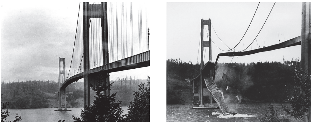
Figure 1.1: The Tacoma Narrows Bridge before (left) and after the collapse (right) (picture courtesy: University of Washington Libraries, Special Collections).
